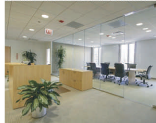
LAY IN METAL TILES & GRID
