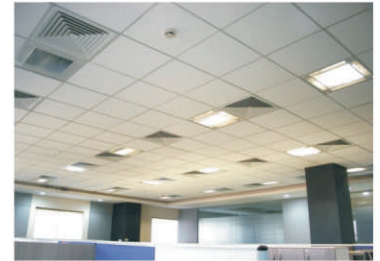
GRID + GYP TILES FALSE CEILINGS
