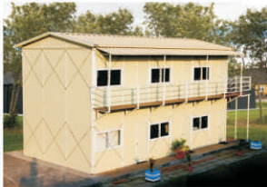
PRE ENGINEERED ACCOMMODATION
