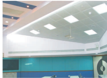
GYPSUM + METAL FC IN SLOPE & STEPS
